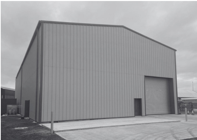
Diffusion Alloys (UK) Ltd, Middlesbrough. Completed 2022
